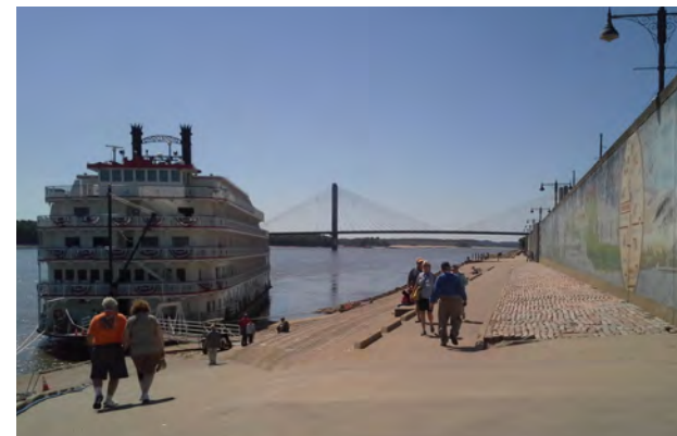
Riverfront area along flood wall
