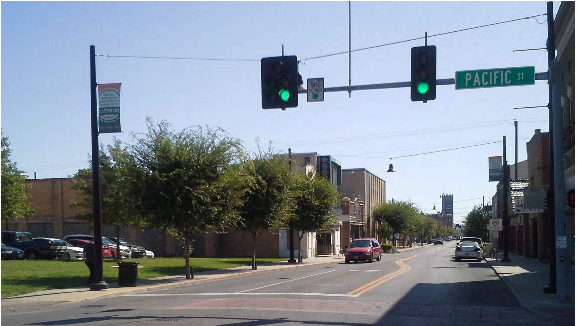
View of the existing conditions at the intersection of Broadway and North Pacific Street. (View to the east.)
